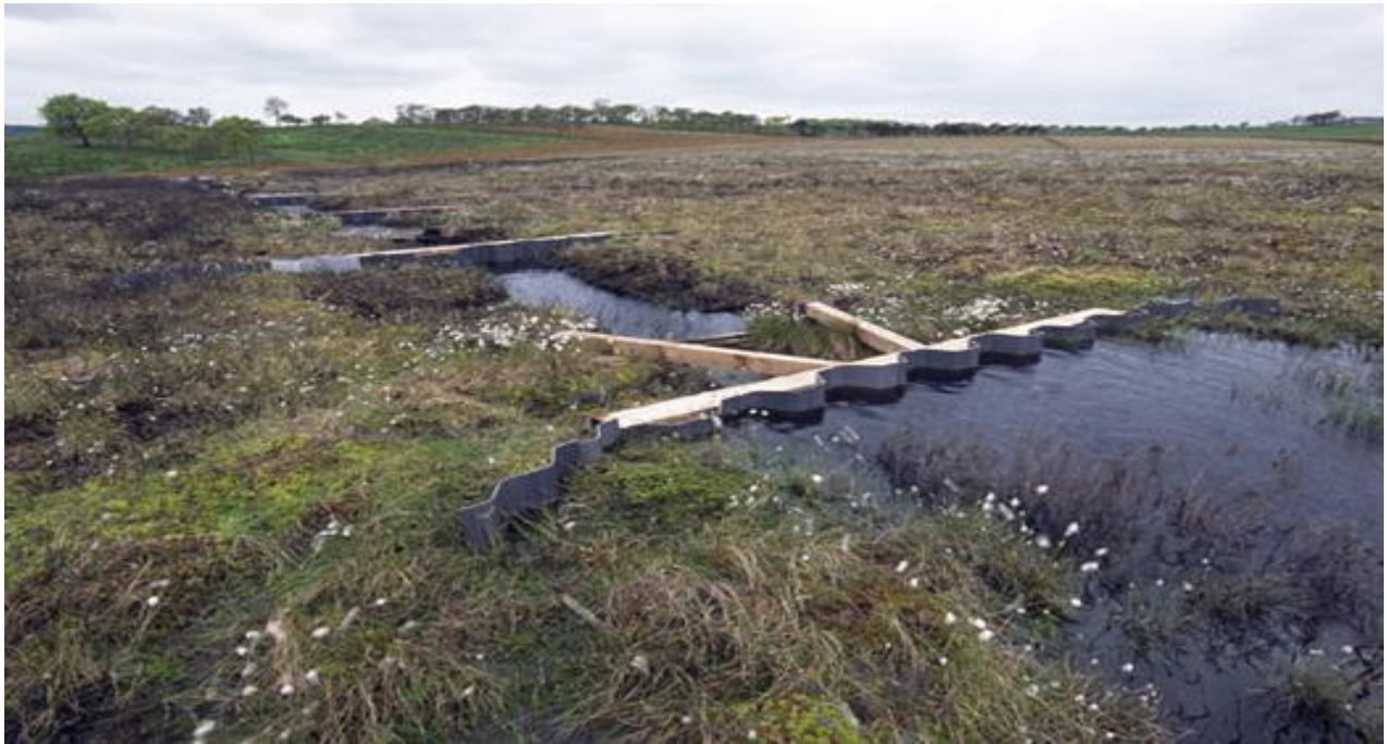
Pic.10 Rehabilitation of the hydrological regime of a raised bog through partitioning off the drainage canals. Blowhorn reserve, Central Scotland
